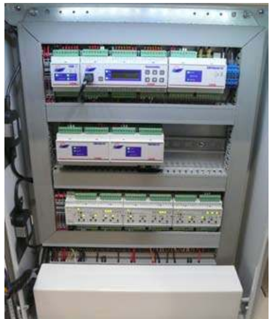
The OEM Foxtrot with the SMS module, CAN-Bus / NMEA2000 Converters and the I/O modules on the CIB bus system.
